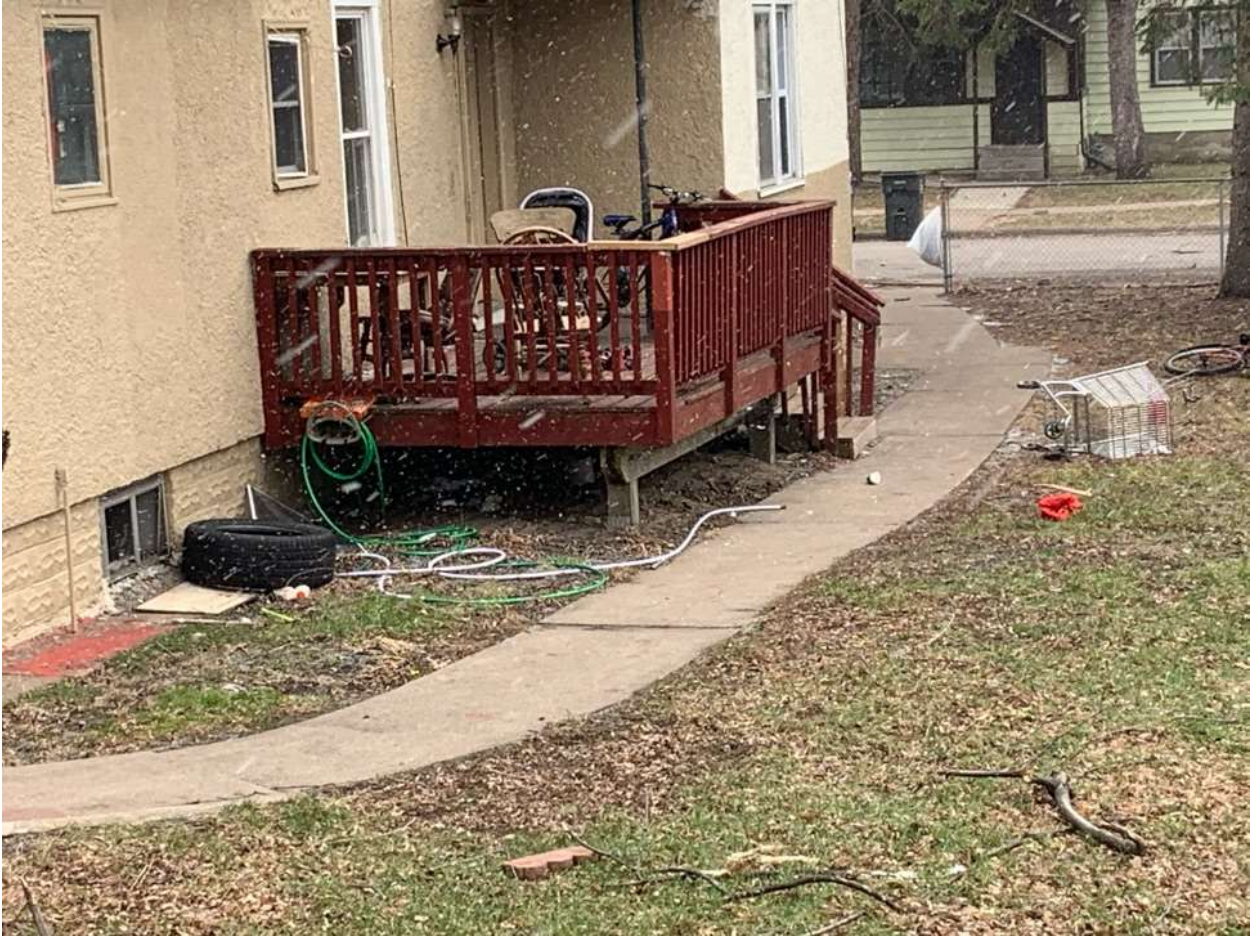
501 Hopkins St Photos rechecked on 4/15/22
