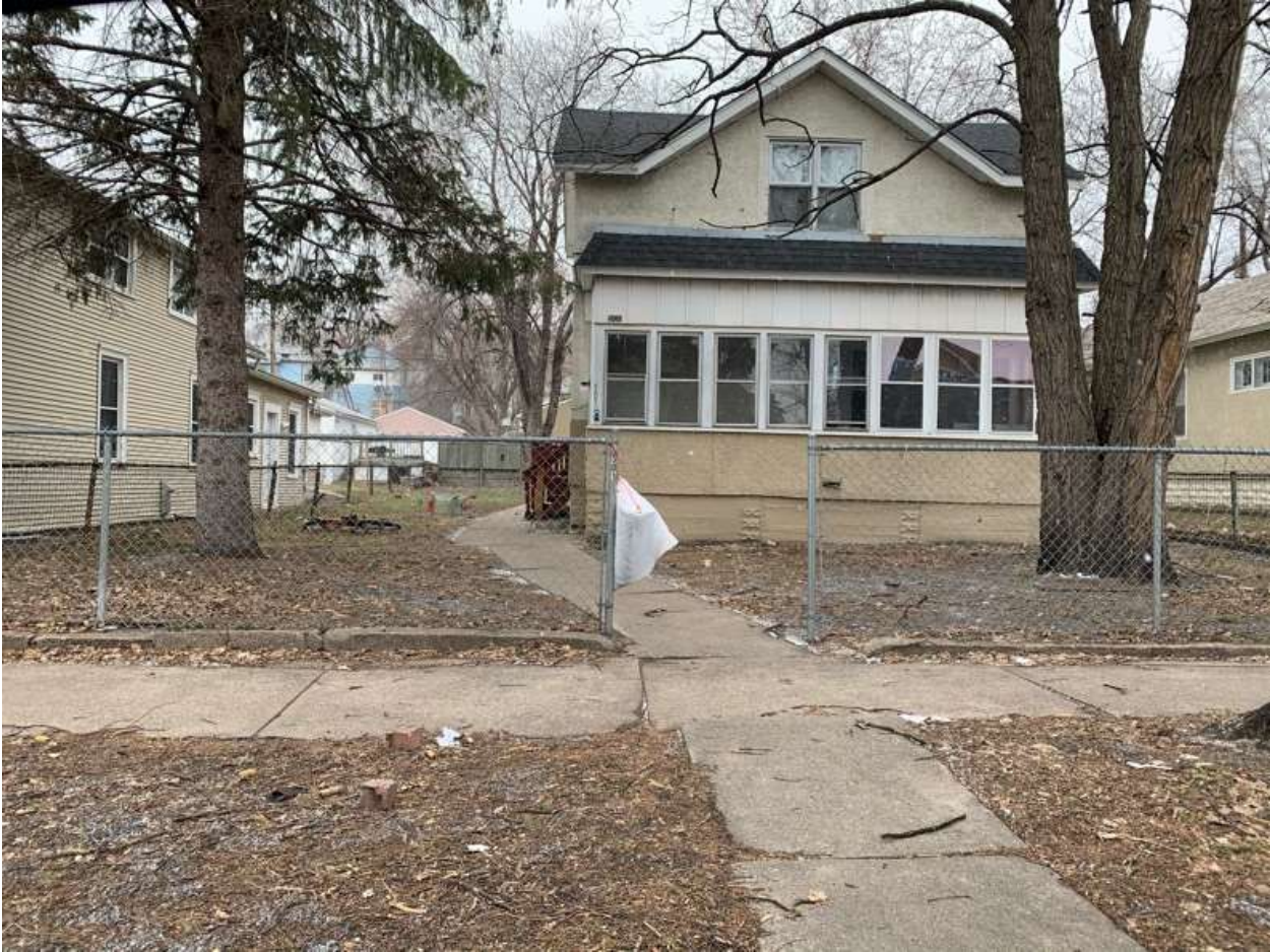
501 Hopkins St Photos rechecked on 4/15/22
